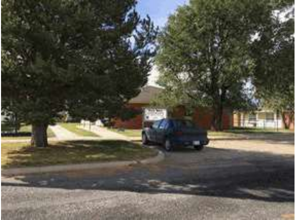
Rent Survey 1 Black Mesa Apartments
