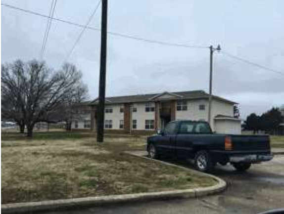
Rent Survey 1 Timberline Apartments aka Wilburton Village Apts
