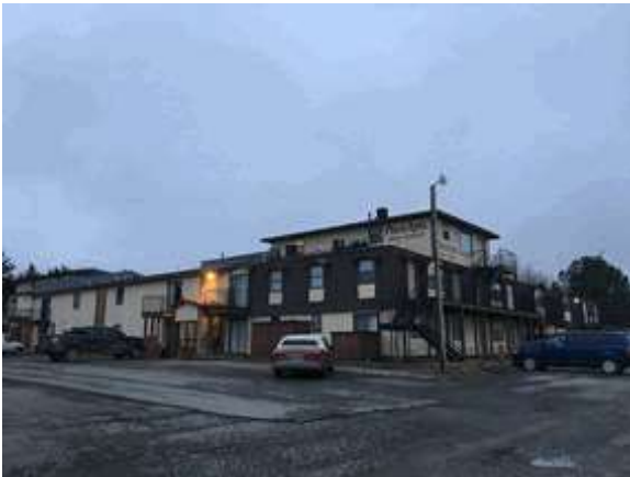
Rent Survey 3 Plaza Apartments
