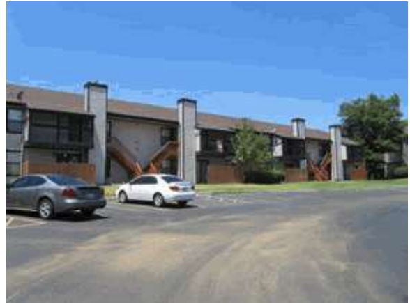
Phoenix Village Apartments
