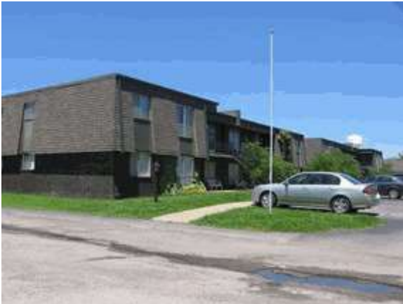
Rent Survey 1 1800 Center Apartments
