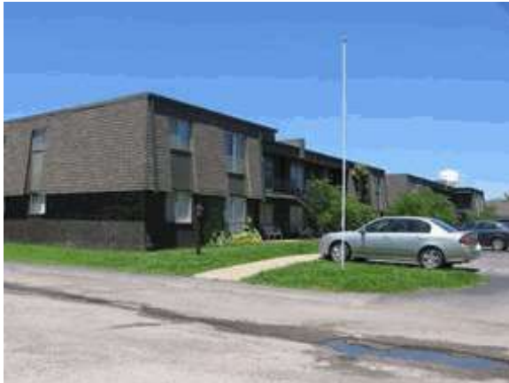
Rent Survey 1 1800 Center Apartments
