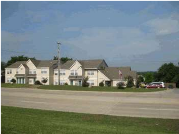
Winding Creek Apartments
